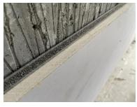
WallArmour dB should be secured onto the wall using 80x6mm hammer fixings. All joints should be staggered. Starting in the bottom left-hand corner of the wall, offer a board up to the wall, resting the panel on 5mm spacers at the floor junction and against some 5mm
