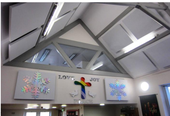
All Saints Primary School, Kirkby Overblow, North Yorks
