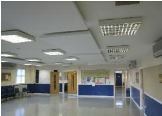
Sonata Vario absorbers fixed to a ceiling.
