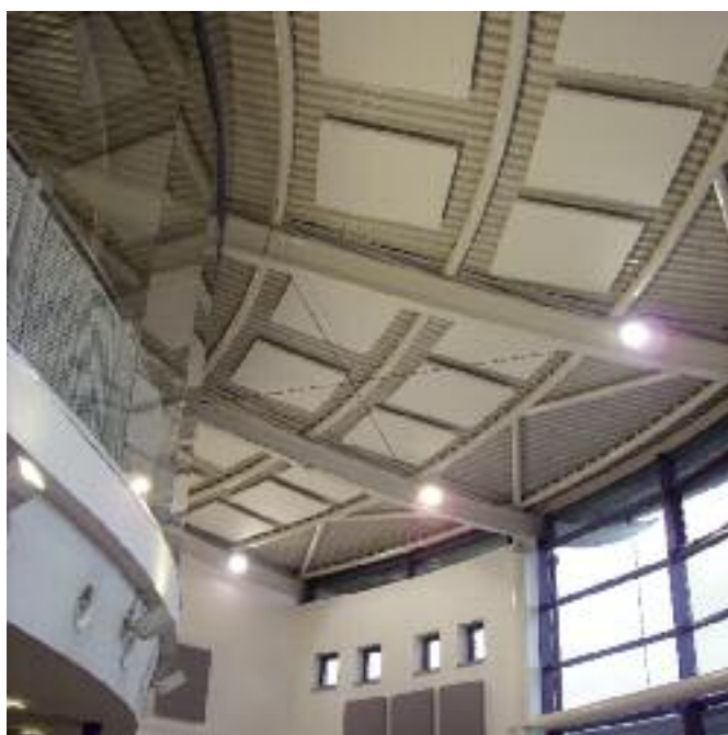
Sonata Vario installed on a ceiling
